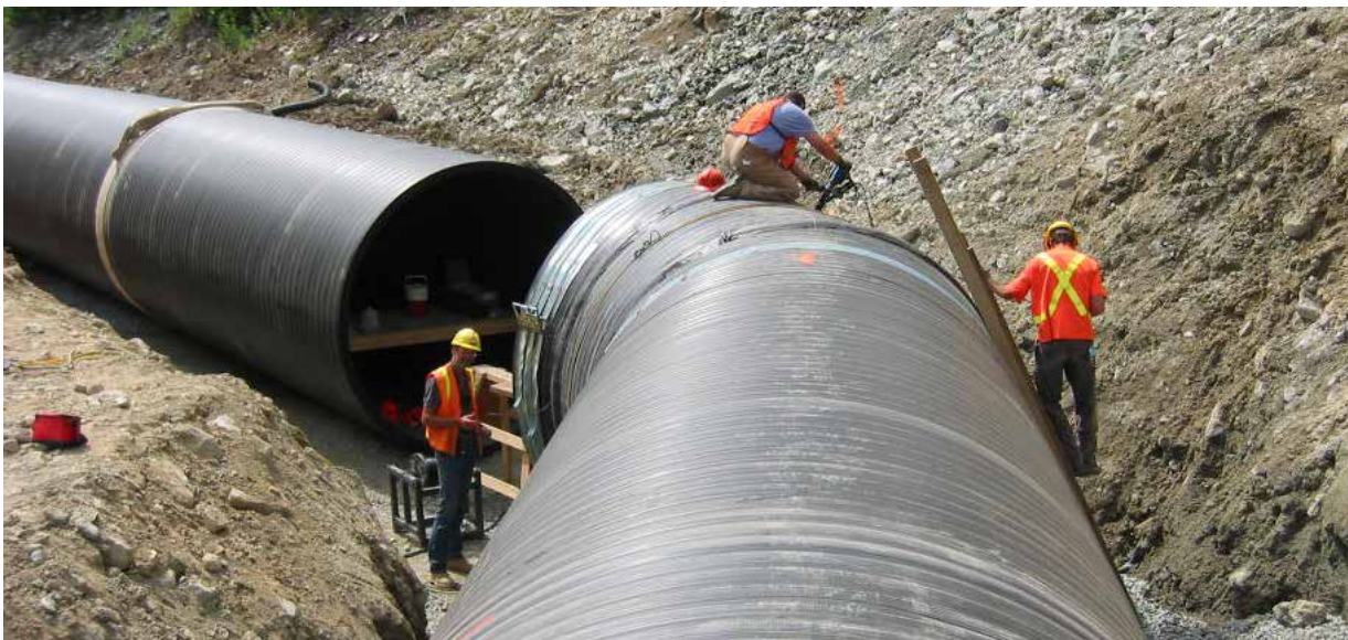
FIGURE 4.20: STRUCTURED WALL HIGH DENSITY POLYETHYLENE
