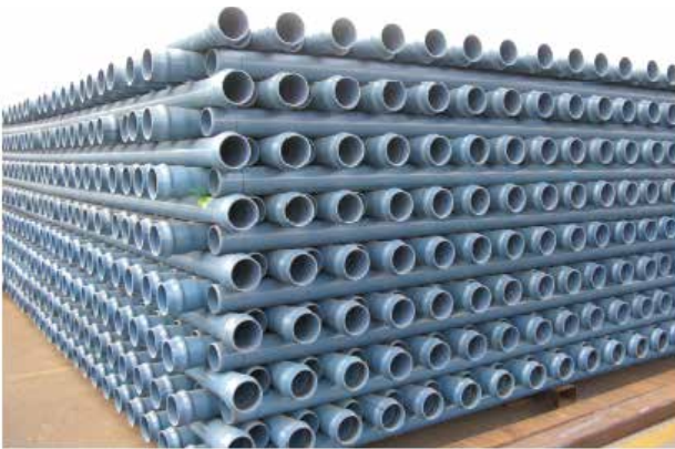
FIGURE 6.1: STACKING OF PVC PIPES
