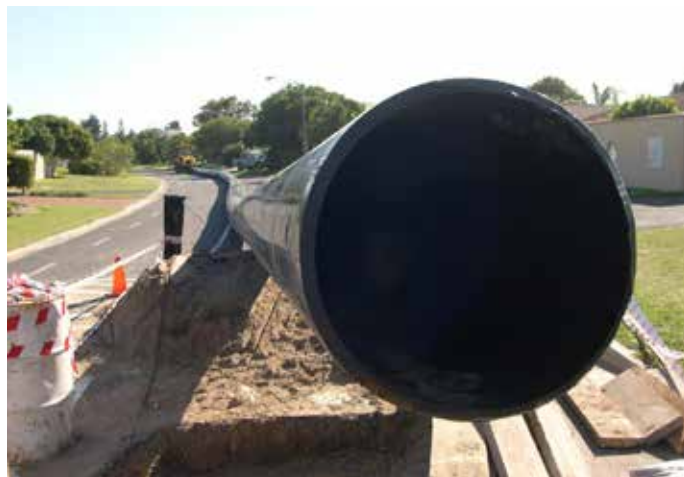
FIGURE 6.12: SLIP LINING
