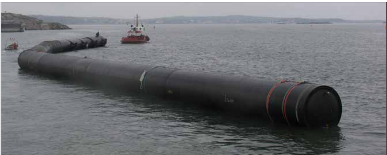
FIGURE 4.21: STRUCTURED WALL PE-HD FLOATING SYSTEM
